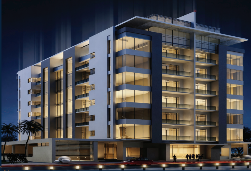
G+6 CONSTRUCTED IN 2015 - 2016 IN AL WARQA AREA, DUBAI
